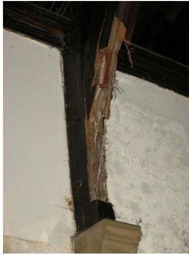
Dry Rot in a Roof Beam
