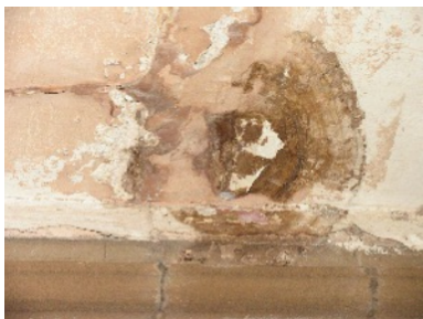
DRY ROT INFLORESCENCE
