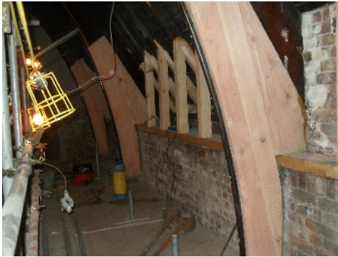
BEAM REPLACEMENT CHANCEL ROOF
