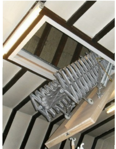
ACCESS TO CHANCEL ROOF LADDER
