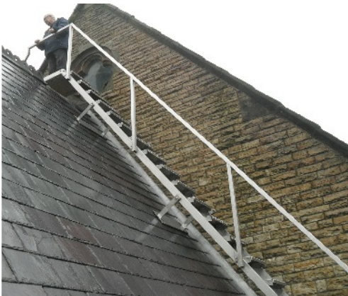
CHANCEL ROOF LADDER
