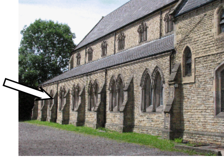
South Side Showing the Clerestory Windows and South Door
