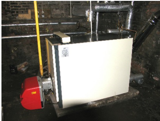
The New Boiler
